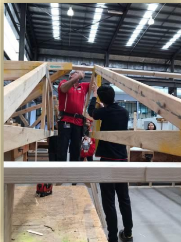
屋頂木桁架組裝-2
