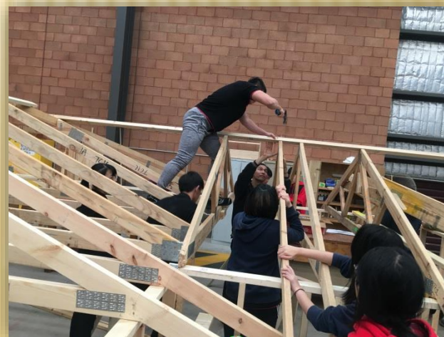
屋頂木桁架組裝-5
