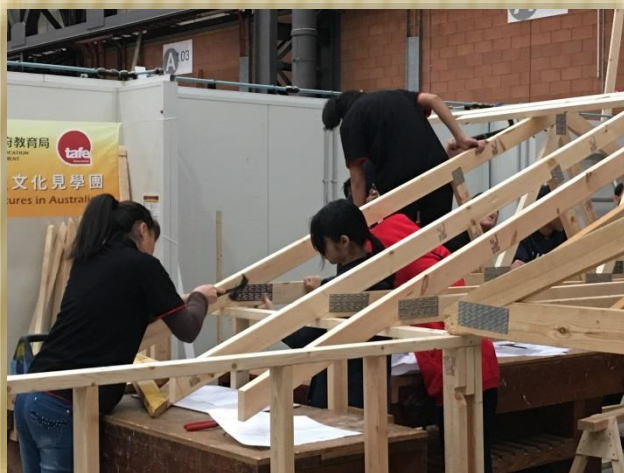
屋頂木桁架組裝-4
